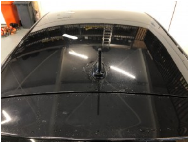
Roof - Hail damage
