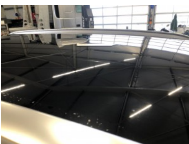
Roof - Restyle dent
