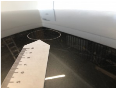
Roof - Restyle dent
